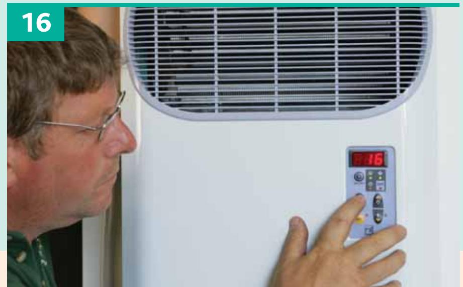
Plug in motor and set controls. See manual with motor. Please note that the fan motor runs continually.
