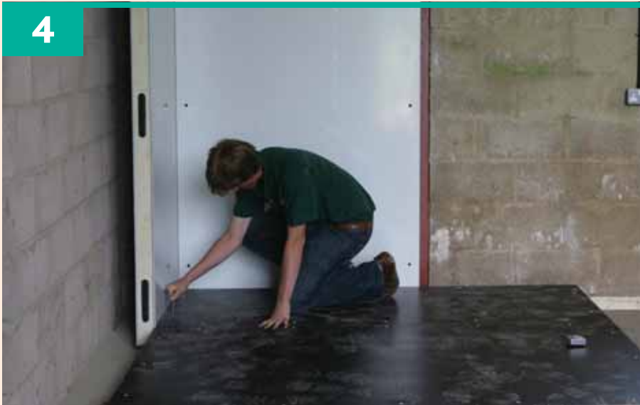
4 Fit corner wall panels. Please note wall panels have three cam locks, ceiling panels have more.
