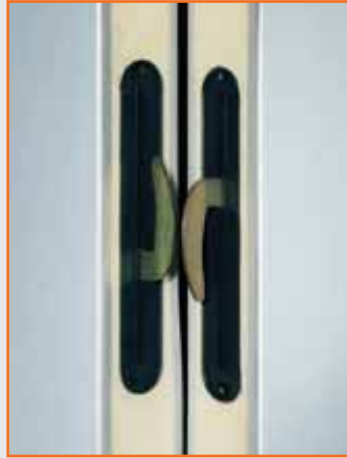
Panels are joined together with cam locks.
