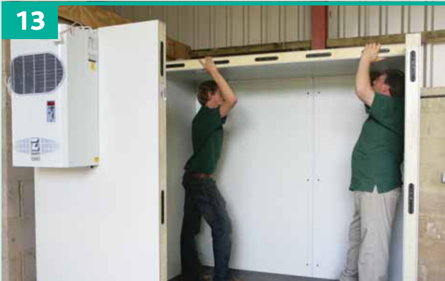
Fit ceiling panels.
