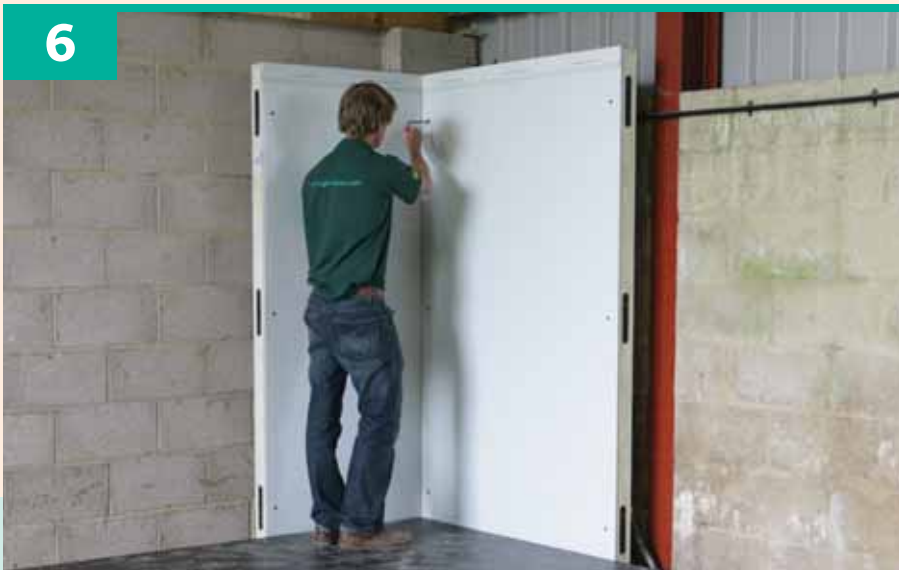
4 Fit corner wall panels. Please note wall panels have three cam locks, ceiling panels have more.
